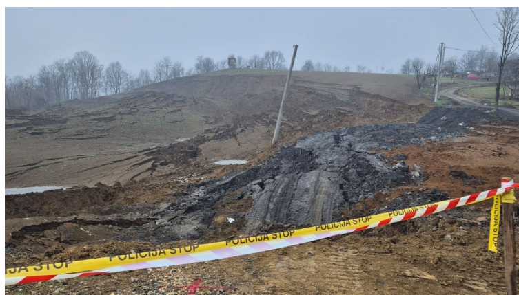
Figure 8 - "Strupina" landslide near Maglaj city
