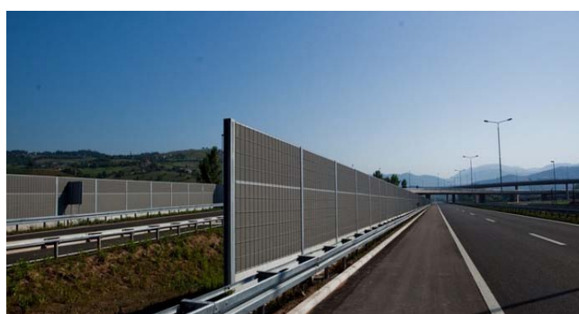
Figure 6 – Barriers for protection against noise
