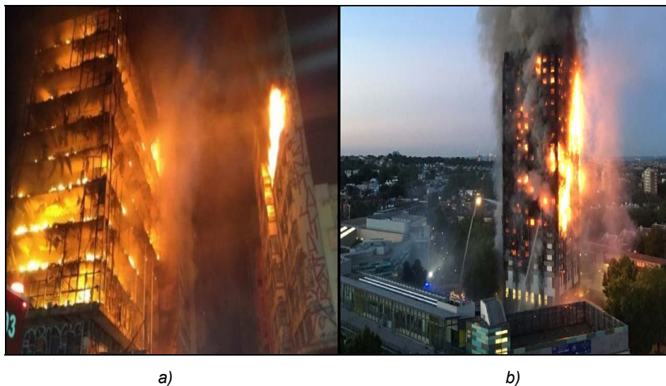
Figure 1 – Huge fire in a residential building in Sao Paolo, Brazil, in 2018 (a) (Fos Media, 2018) and a huge fire in the residential building Grenfell Tower in London, UK, in 2017 (b) (Hartley-Parkinson, 2019)
