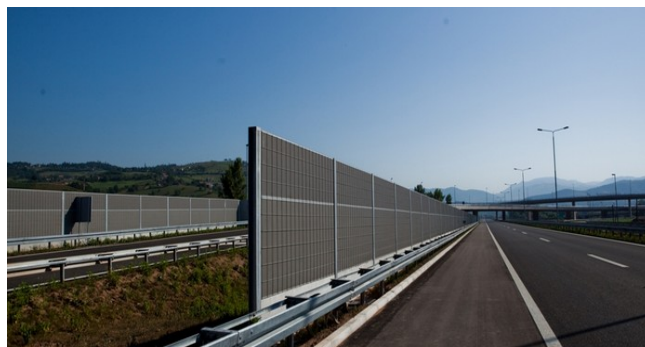
Figure 6 – Barriers for protection against noise
